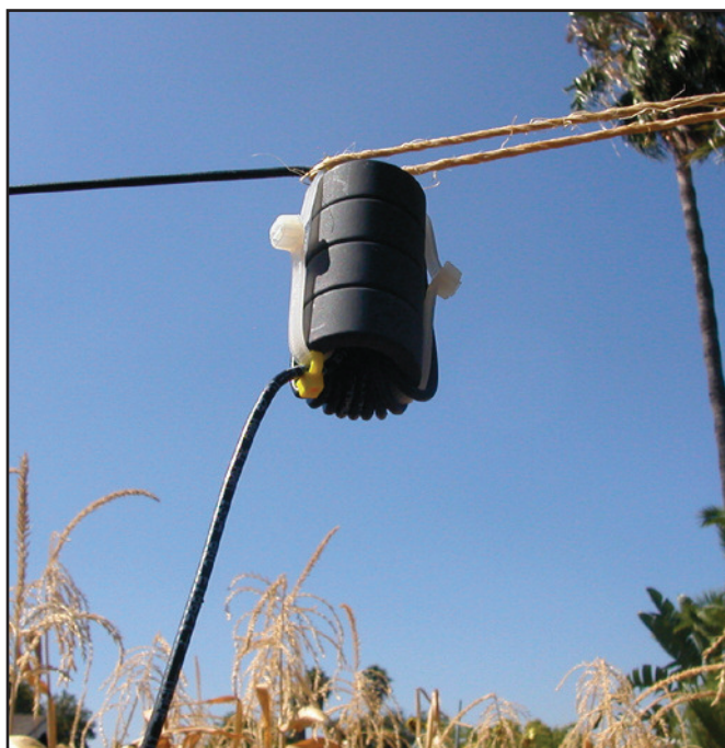
A piece of string was used at the RF choke point of the RG-174U coax to tie-off the EFD about four-feet above the ground. Non-resonant coax leading from the bottom of the toroid stack goes to the transceiver or tuner.
